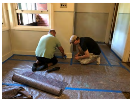
Internal repairs being undertaken at Calthorpes' House
