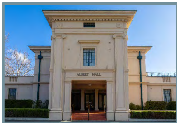
Exterior view of the Albert Hall.
